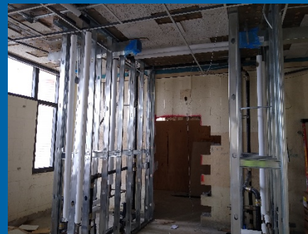
Installation of Overhead Pipes and Pipe Insulation in Building 2010
