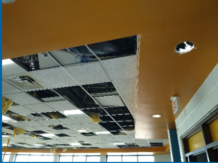
Continue Install of New Lighting in Media Center
