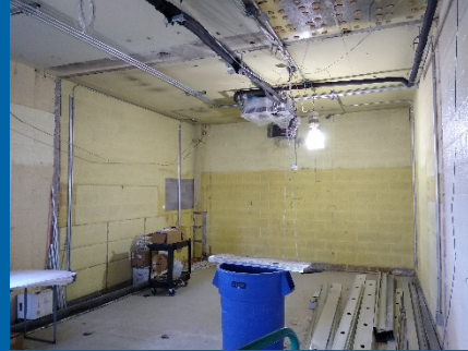
Install Conduit in Administrative Area of Bldg 2010
