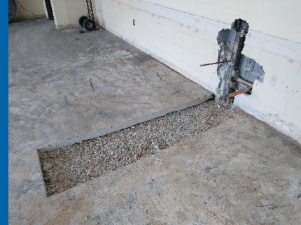
Relocation of Water Supply Line in Art Room
